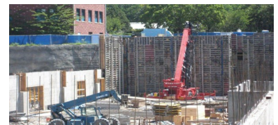
Recent Project from Iron Eagle’s Delta Mechanical Subsidiary
